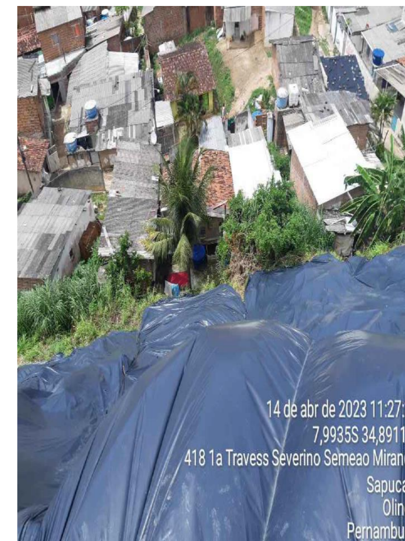
RUA SEVERINO MIRANDA - R$ 2.449.043,34
