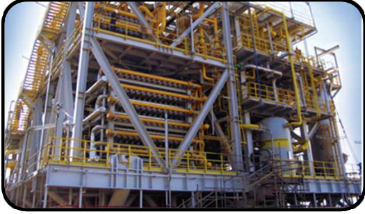
First CO2 separation from associated natural gas in ultra-deep water
