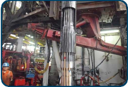
First intensive use of intelligent completion in ultra-deep water
