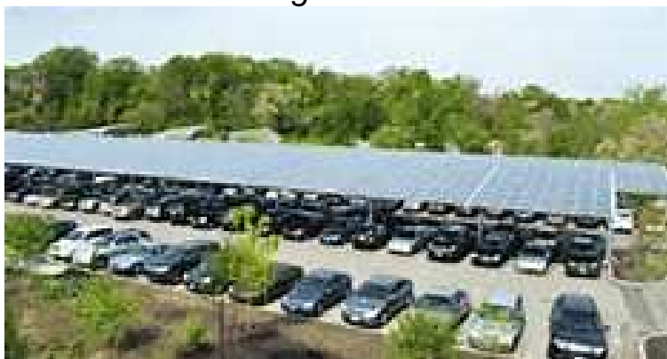
Parking lot Sheds
