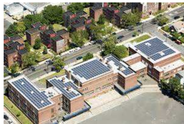
Roof top Solar Panels
